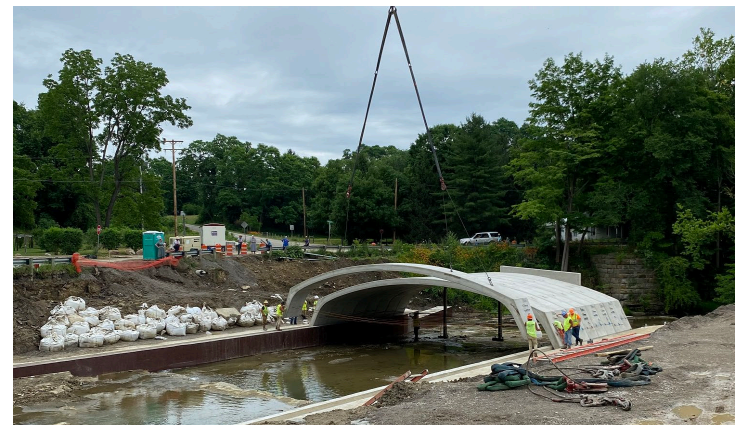
Setting the arches for Bundysburg Road Bridge on 7/22/2022
